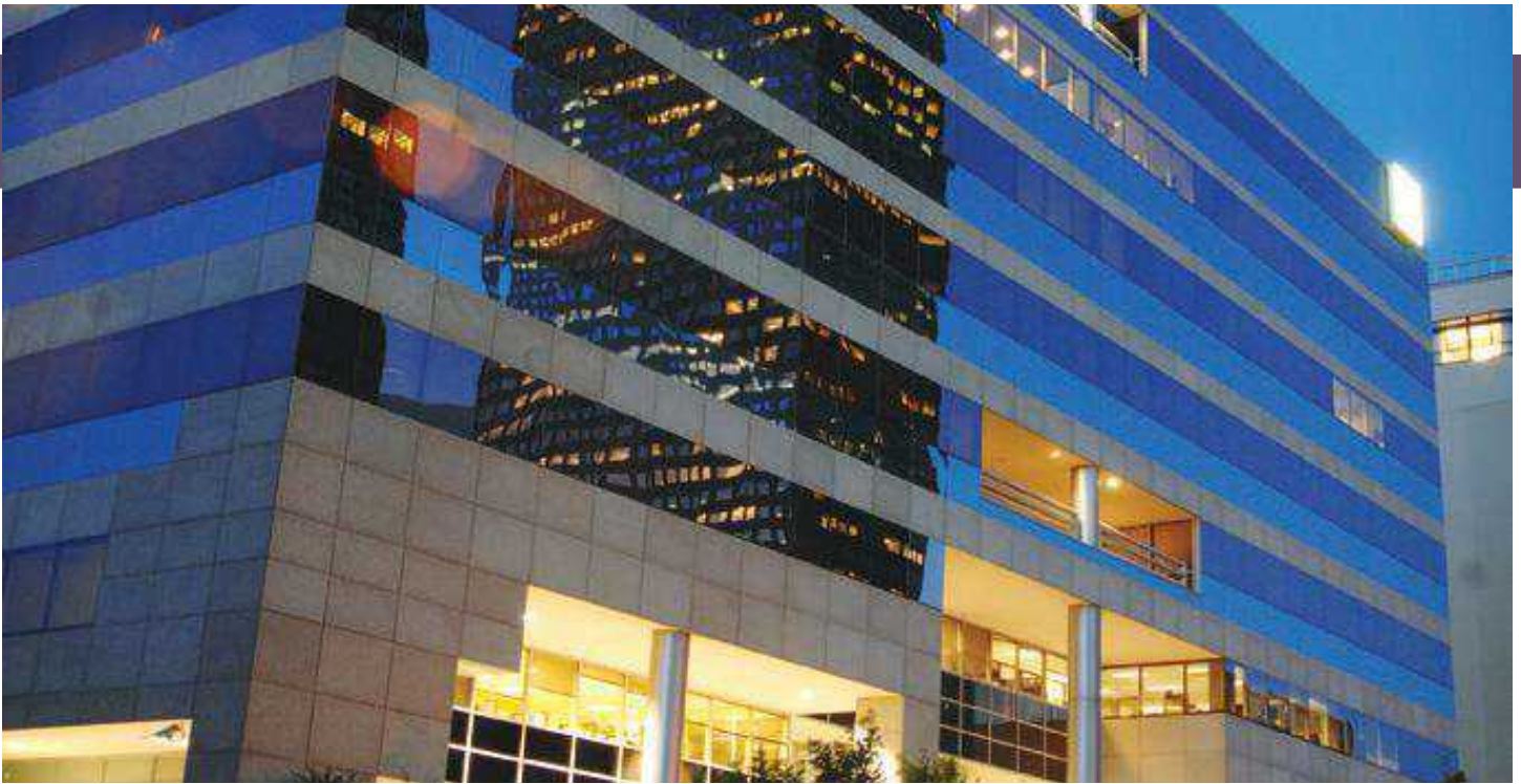
The University of Colorado's headquarters at 1800 Grant St. in Denver.
